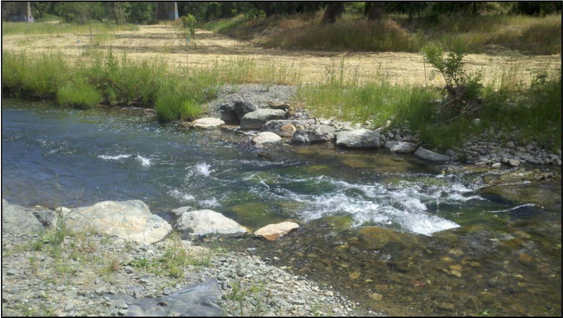
Cross-vane structure at Putah Creek. Note convergent flow center channel.
