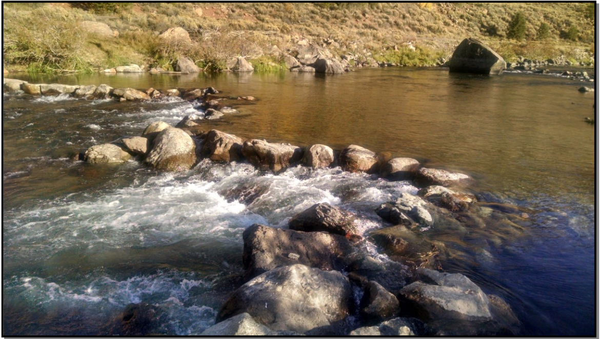
Boulder W-Weir on Truckee River. 2017 Photo
